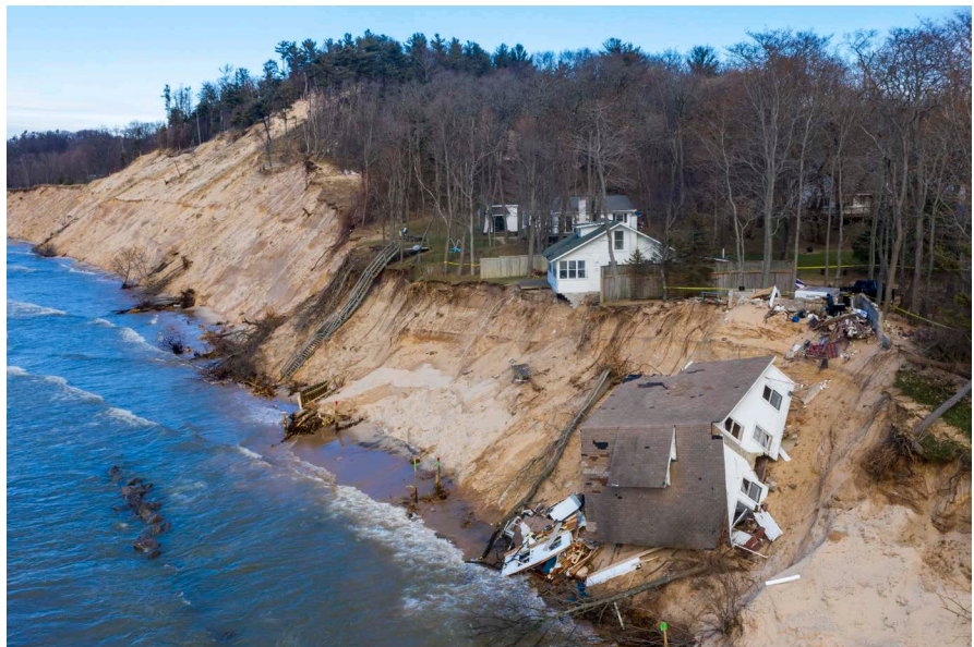
Figure 24. Lake Michigan erosion claims a beach house on January 2, 2020, in White River Township, near Montague, MI © 2020 Mlive Media Group. All rights reserved. Used with copyright permission from JWARP [5].
