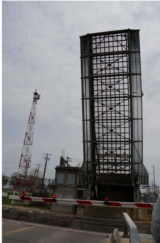
Figure 17. Raised Road Bridge to allow tall ships to pass through the Welland Canal.
