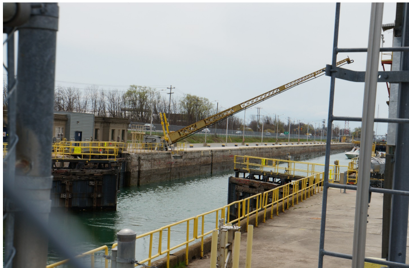
Figure 12. Welland lock with gates open.
