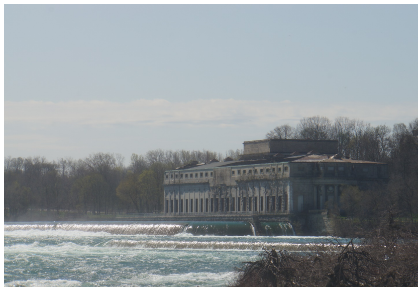
Figure 8. Canadian hydroelectric power plant on Niagara River above Niagara Falls.
