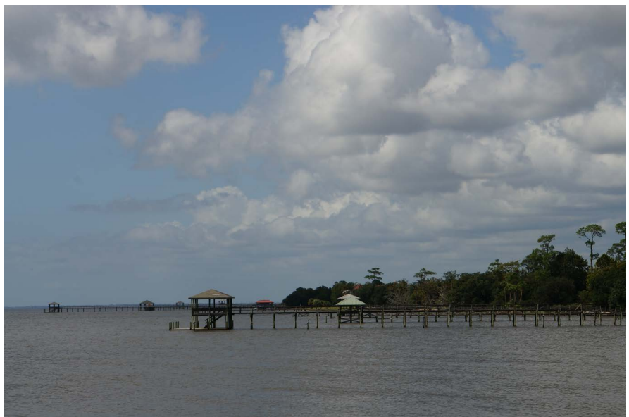
Figure 18. Picture of area piers along the Gulf of Mexico with coastal erosion.
