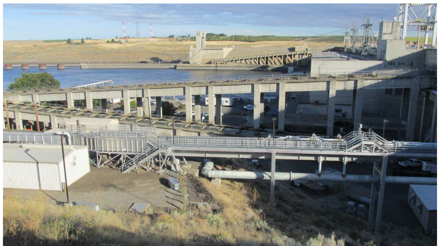
Figure 19. The Ice Harbor dam with a fish ladder on the Snake River just east of the confluence of the Columbia and the Snake Rivers.
