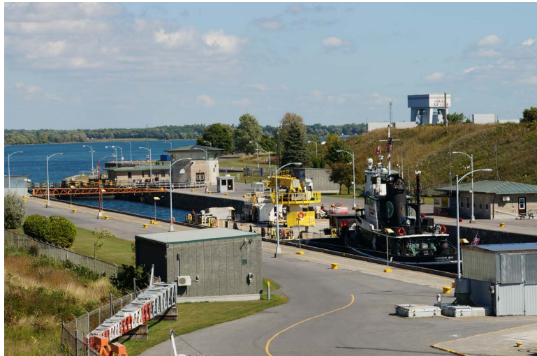
Figure 3. The Iroquois lock and control dam which controls the level of Lake Ontario. Picture taken by Lois Wright Morton.
